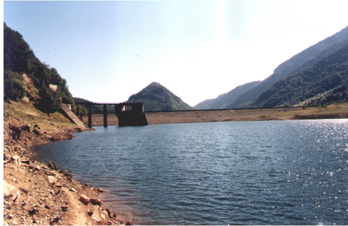
Figure 1. General view of the Motru dam from upstream
