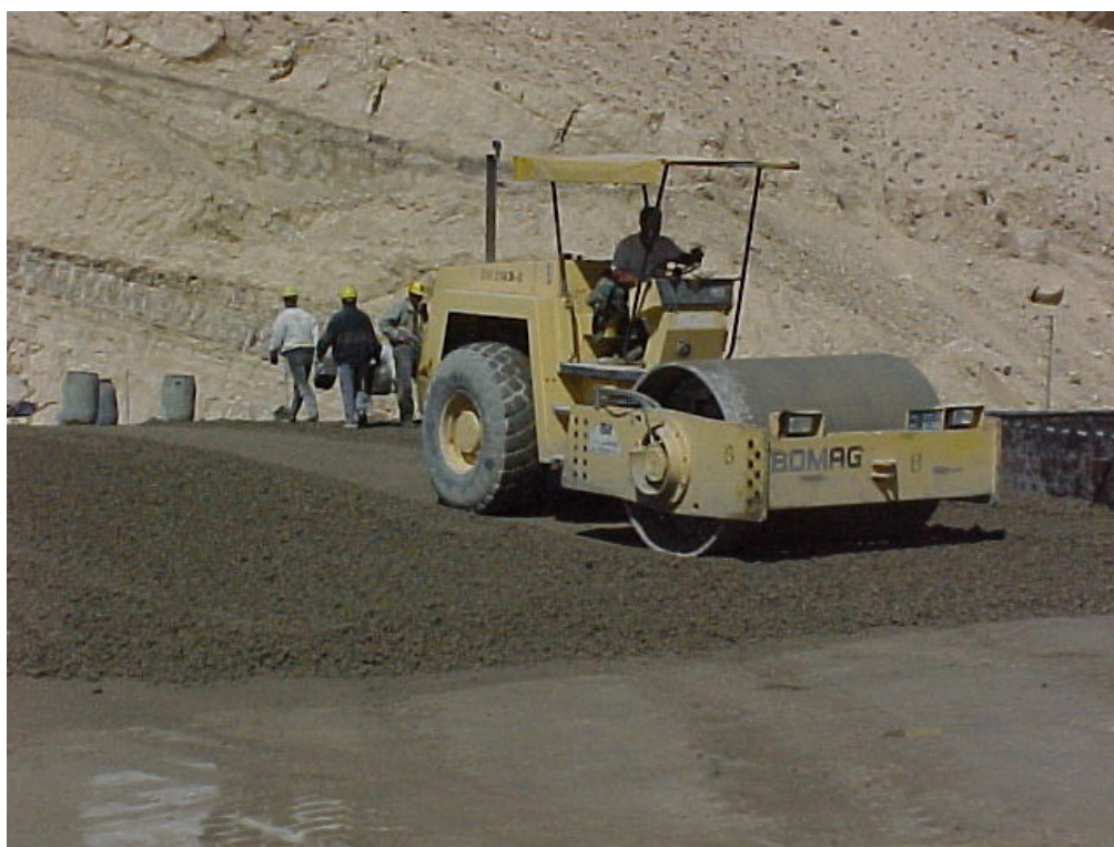
Roller compacted concrete
