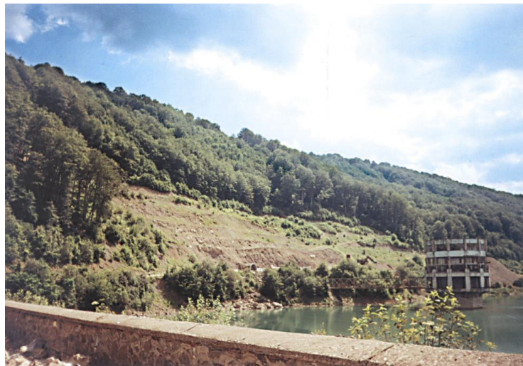
Figure 2. Sacele Dam intake on the right bank affected by slope instability
