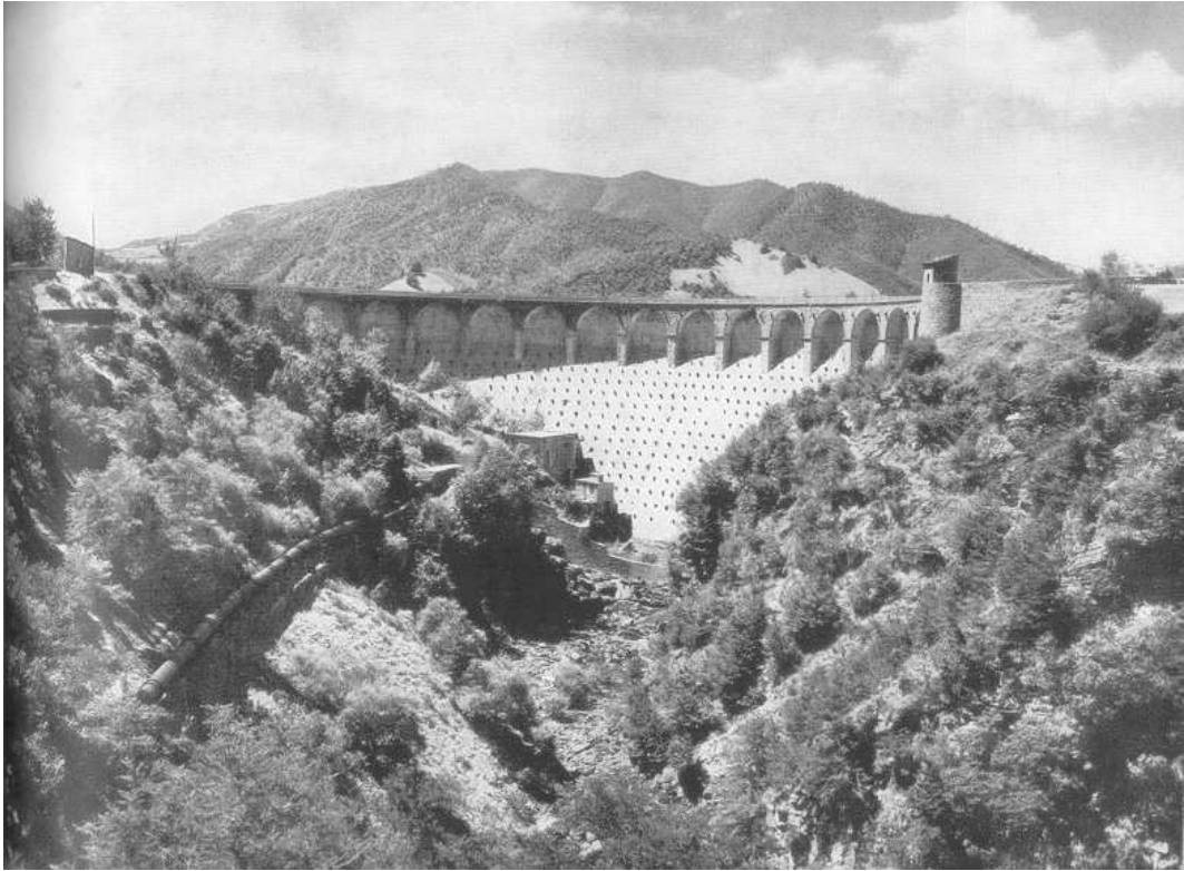
Fig. 1 Downstream view of Scalere dam
