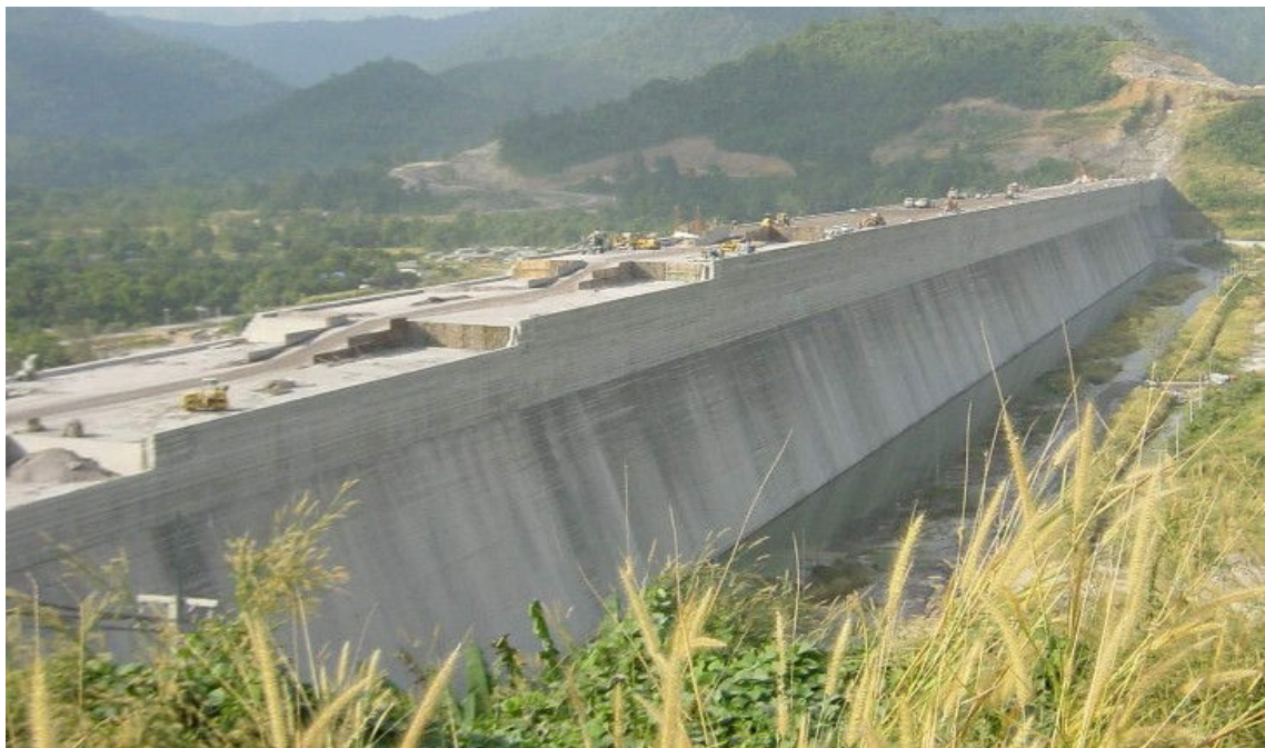
Figure 6 - Thadan RCC dam under construction (end 2002)
