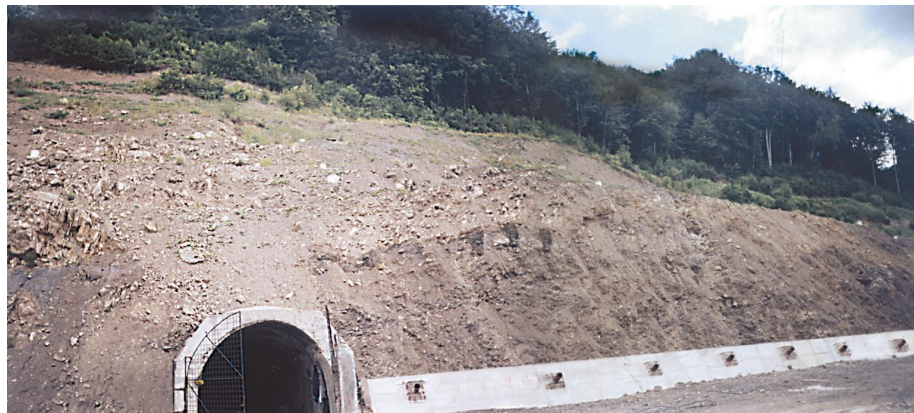
Figure 5. Drainage tunnel portal and the first row of anchors
