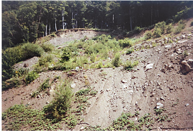
Figure 4. Retrogressive instability induced by the slope reshaping
