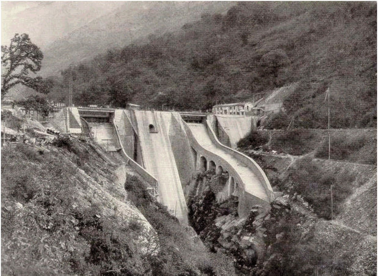
Fig. 1 Downstream view of Poglia Dam
