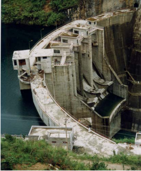
RCC Arch Dam of Puding hydropower station
