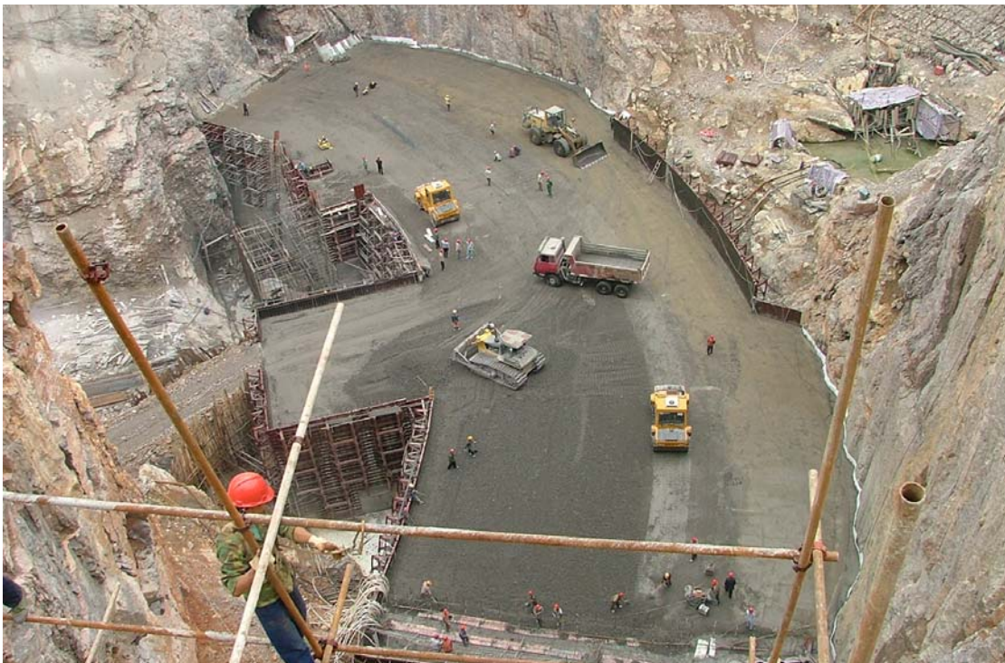
Constructing RCC Arch Dam
