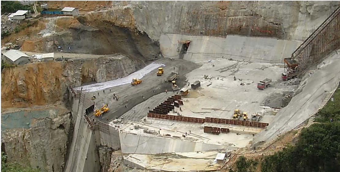
Constructing Left bank Rcc Gravity Dam Cushion Concrete
