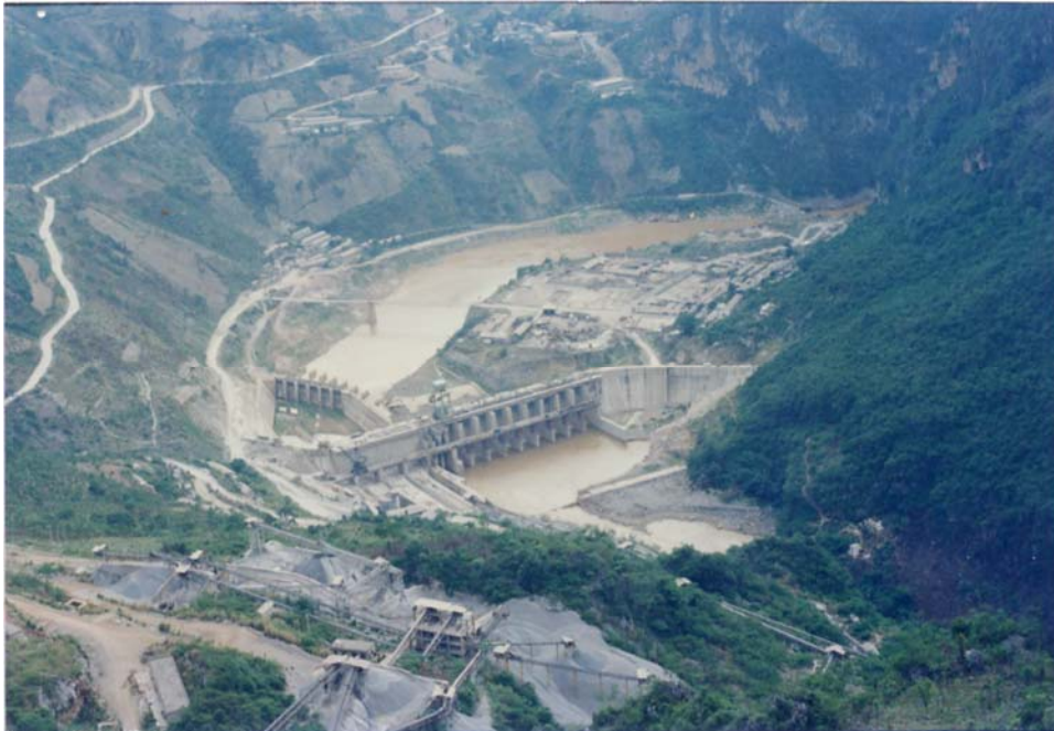
THE TIANSHENGQIAO SECOND CASCADE HYDROPOWER STATION IN GUIZHOU PROVINCE
