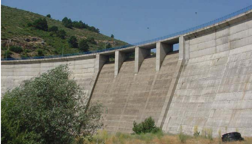
Picture of the Dam
