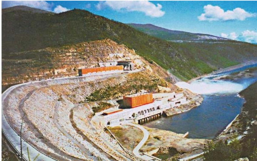
Fig. 1. Kolymskaya dam. Aerial view of downstream shoulder
