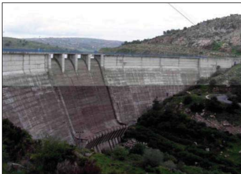
Figure 1. View Of The Dam (From Downstream)
