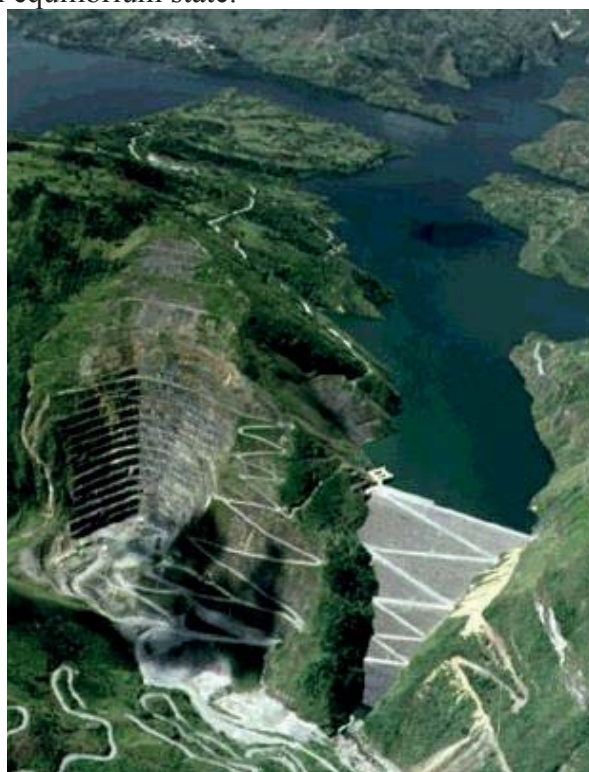
Figure 1: View of the Alberto Lleras Dam
