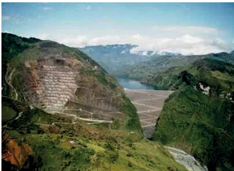
Figure 1: General view of the Guavio Hydroelectric Project and the Alberto Lleras Dam [4]
