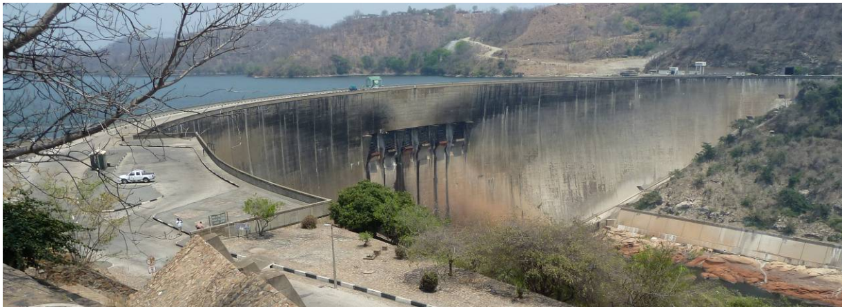
Photo 2: Kariba dam from Right Bank
