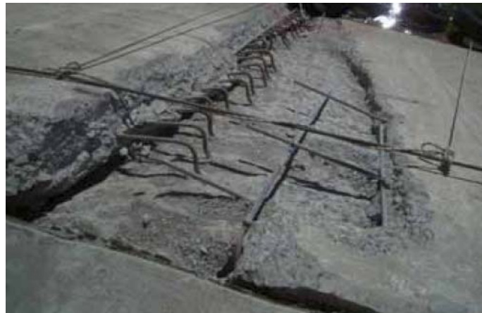
Figure 2: Slabs 17 and 18 after removing sheared concrete
