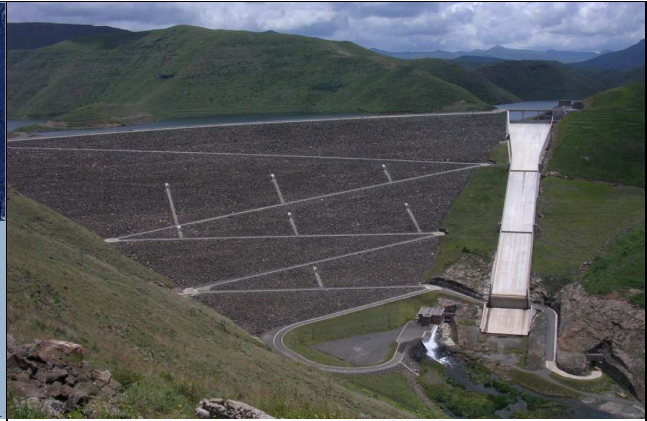
Figure 3: Mohale dam seen from downstream on Dec 24, 2004 1
