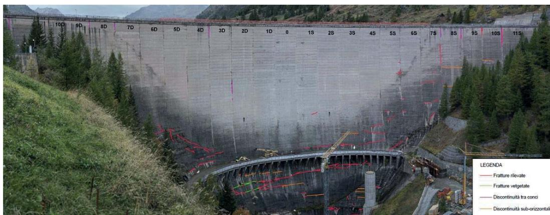
Figure 5: The dam was observed to deflect upstream with cracks appearing on the downstream face and openings of some upstream vertical joints
