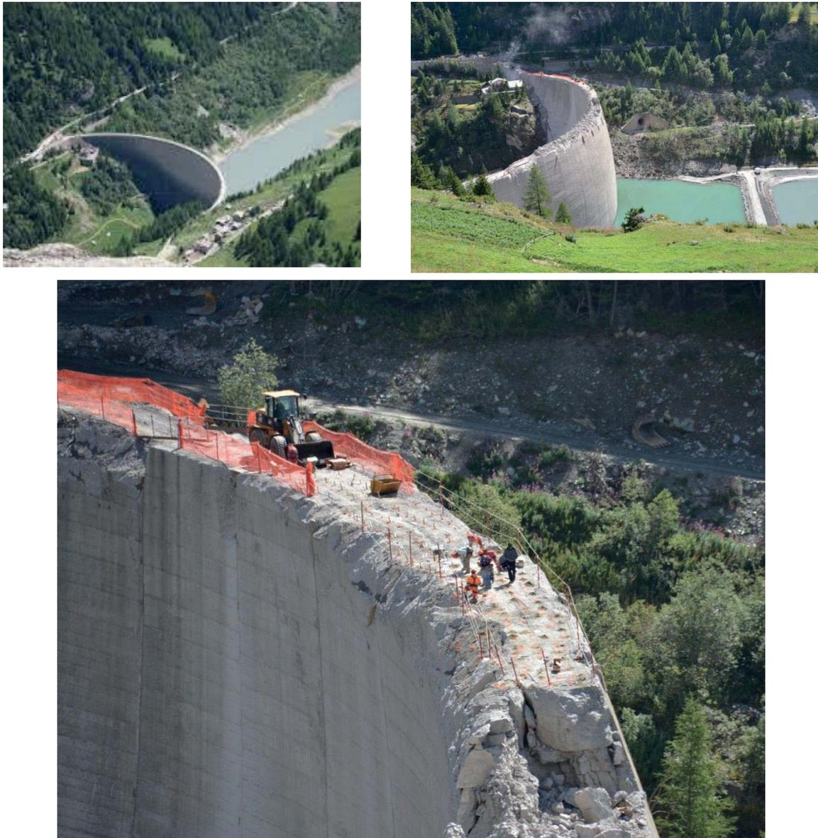
Figure 14: Different sequences of the dam demolition: the dam before the starting of works (up-rigth); the preparation of one explosion step (up-left and down)
