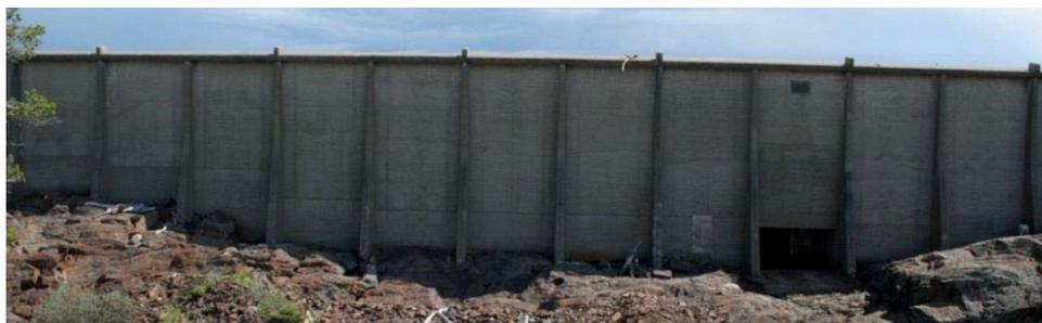
Figure 1: The Håen Dam, view of downstream side with insulating wall
