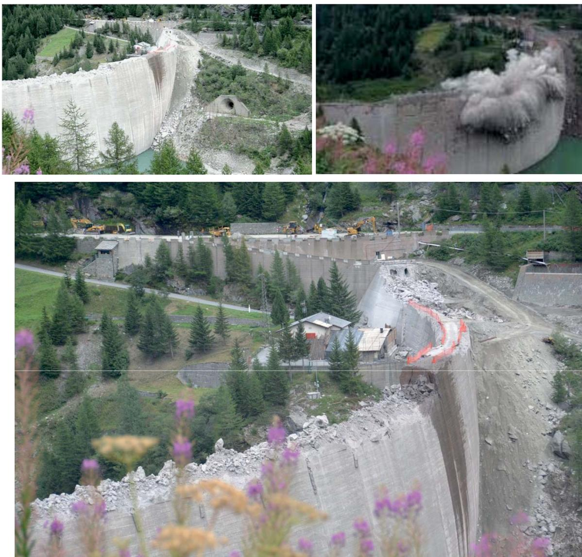
Figure 15: Different sequences of the dam demolition
